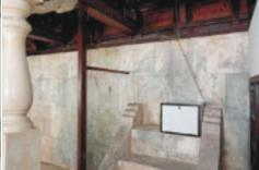
The Coral stone being highly porous and pore diameter being moderately large, the algae had penetrated deep inside the pores, which appeared unsightly. Moreover, the organic acids liberated by the biological growths were further damaging the coral stone.
