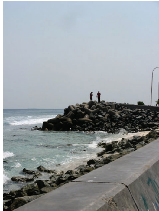
Figure 7. Tetrapod barrier along Male's western coast, bordering land created during the Male' Land Reclamation Project. The tetrapod barriers interlock, and are anchored in coral rubble (blackened by sun exposure and algae) and are backed up by a concrete barrier wall (photo by the author, April 2010).
