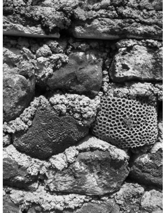
Figure 5. Detail of a typical rough coral wall, likely dating from the late 1980s. Here coral heads were broken into brick-like blocks rather than being used whole ( Porites lutea on the right and likely Platygyra sinensis on the left). This wall rims the municipal dump on Male', in southern landfill created by the Male' Land Reclamation project. In many cases such walls are covered by stucco.
