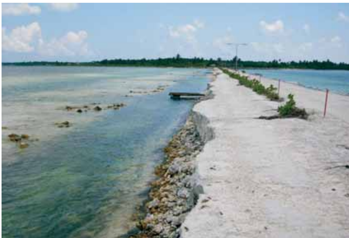
Extensive erosion and scour on western side of the causeway connecting L. Fonadhoo and L. Kaddhoo. Credit: B. Richmond
