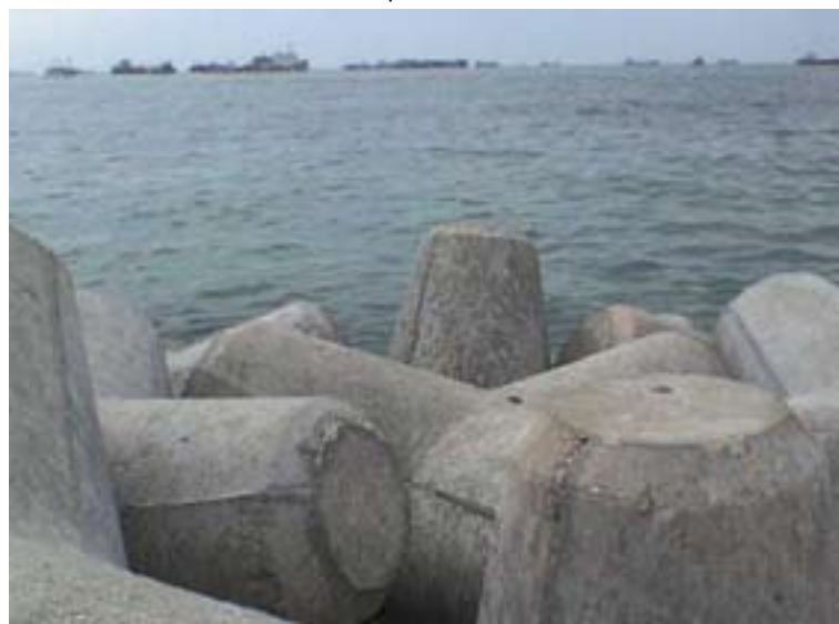
Tetrapod seawall around Male’
